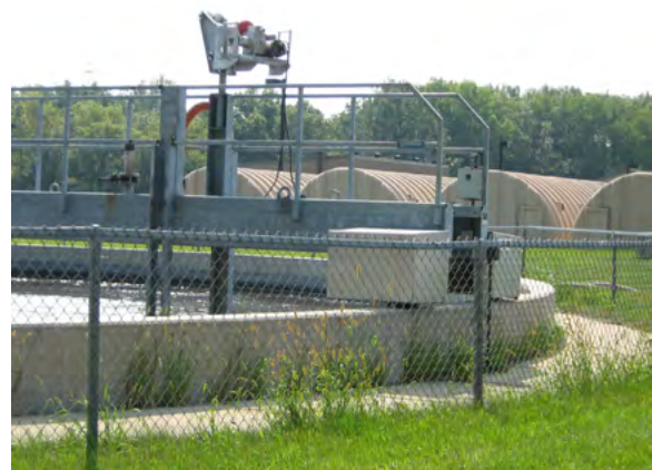
The municipal sewage treatment plant in the Village of Jackson.
