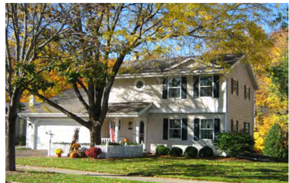
This home is approximately the median age of homes in the County.
