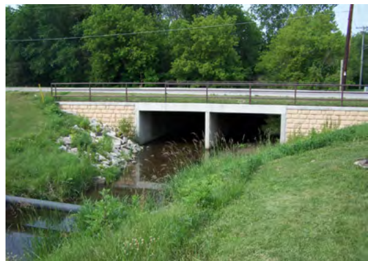
The County currently provides bridge inspection and consultation services to all local governments.
