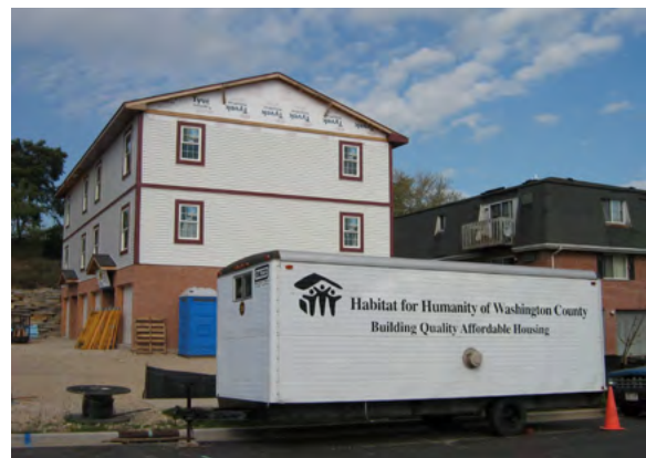
A multifamily home under construction by Habitat for Humanity.
