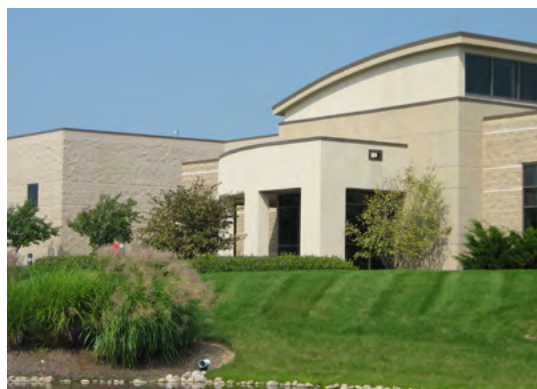
Much of the industrial land in the County is concentrated in business and industrial parks in cities and villages and on the west side of Allenton.
