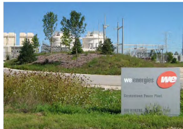
Most of Washington County is provided with electric power service by We Energies.
