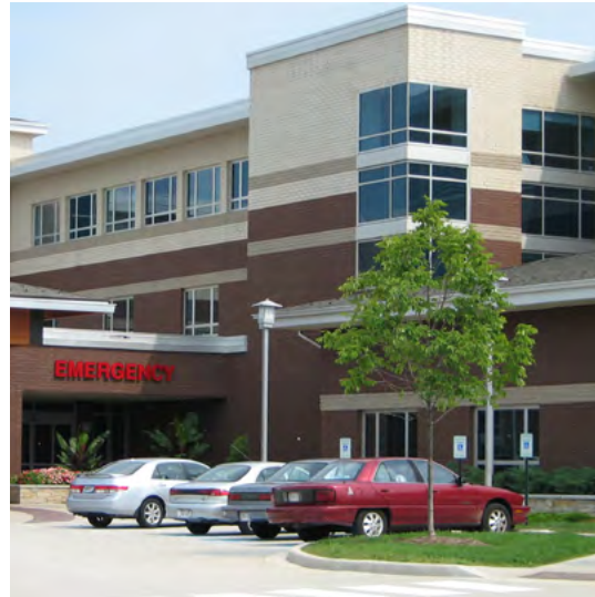
The existing health care facilities in the County were viewed as a strength in the SWOT analysis.
